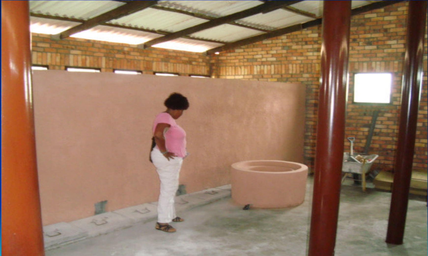
The Digester underneath the Super Structure
